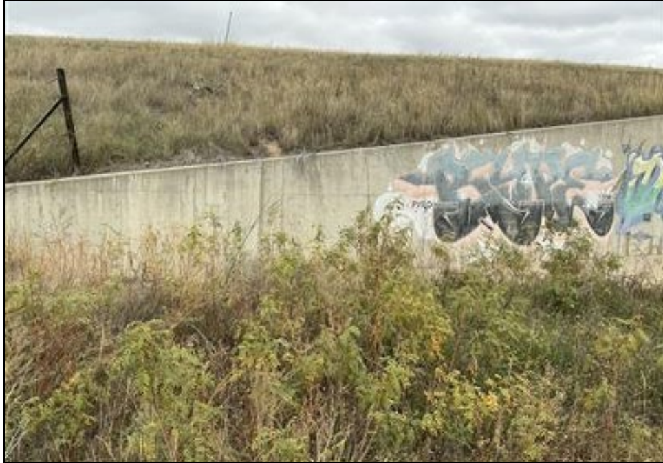
Figure B-13. NDP_01; view facing north
