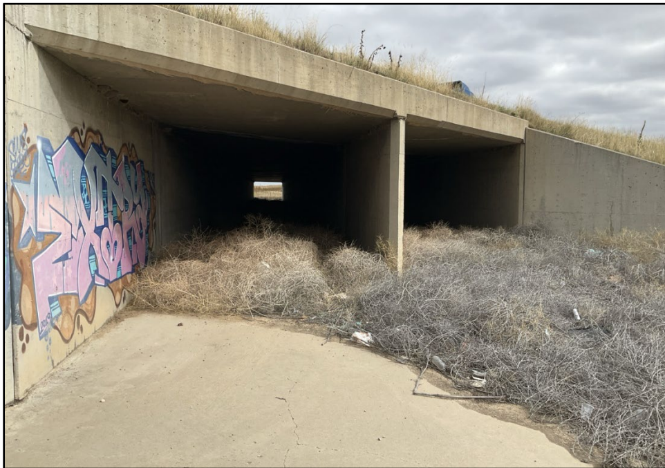
Figure B-24. Culvert northeast of OHWM01; view facing northeast.
