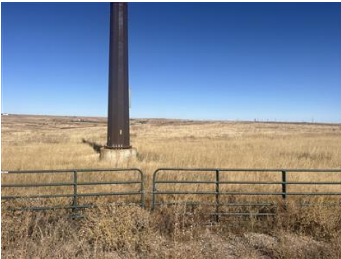
31. Access to STR 593; view facing N.
