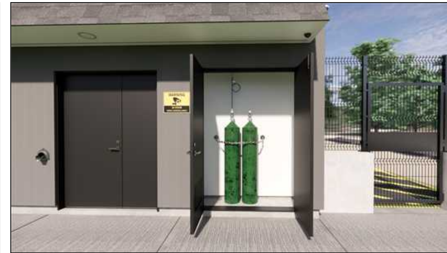
Compressed Gas Enclosure
