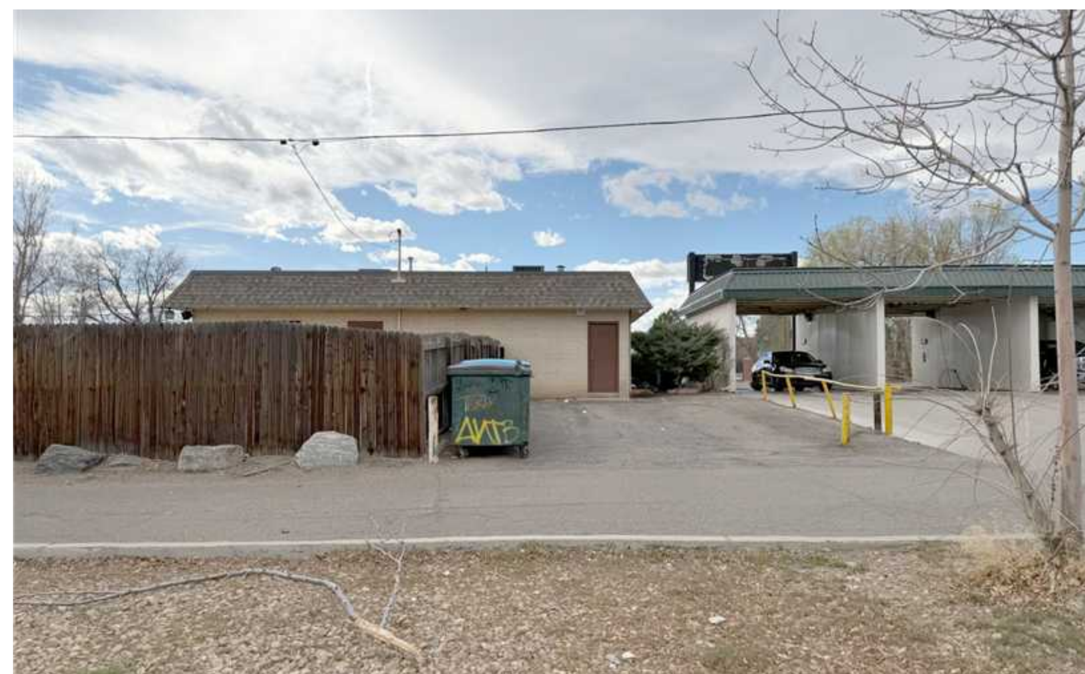
Eastern Existing View
