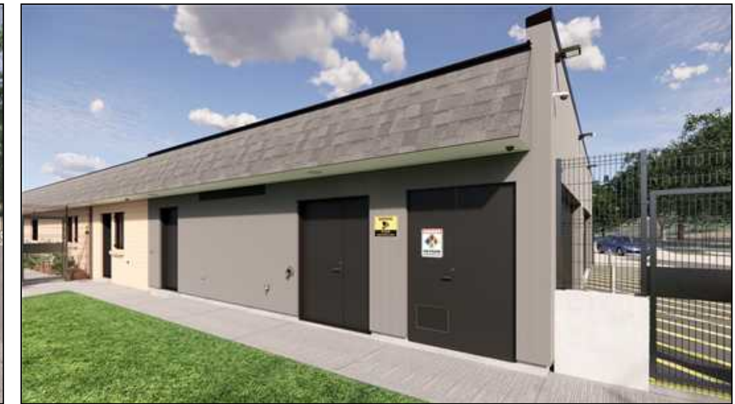
South Facade East Gate, Compressed Gas Enclosure, and Exterior Equipment Roll-Up Door
