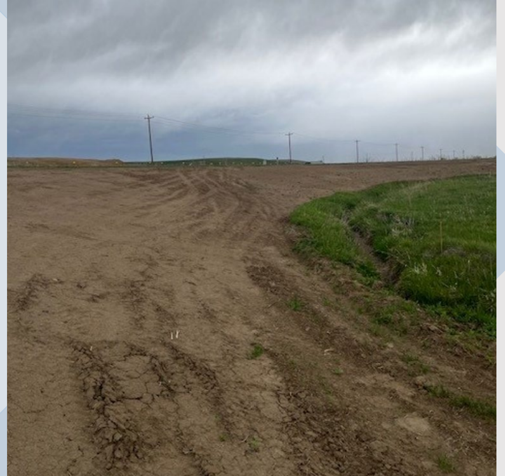
CHANNEL BANK RE-GRADING AND STABLIZATION
