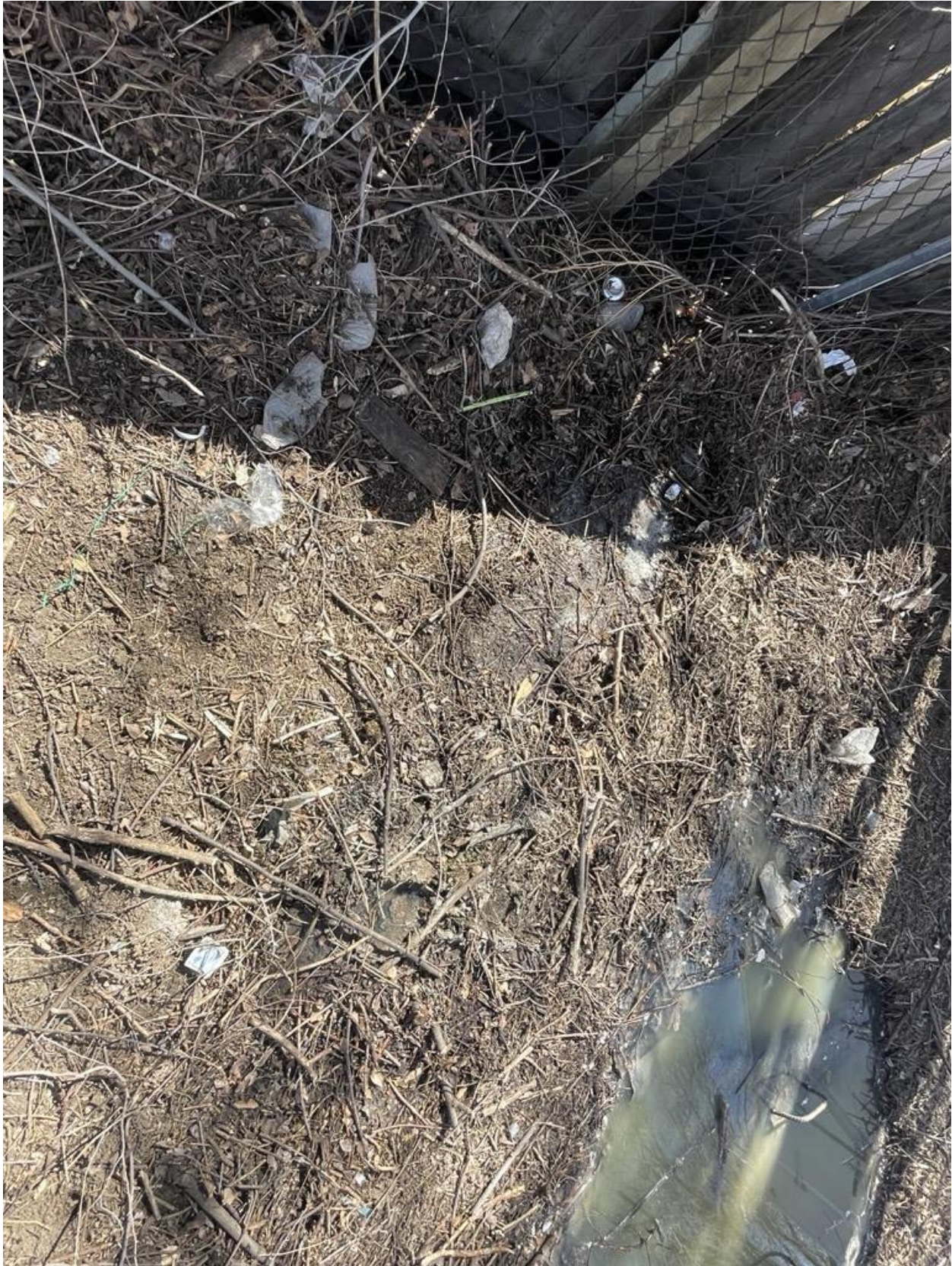
Photo showing proximity (approximately 5 feet) of surfacing effluent to the fence line. Photo angle is looking West
