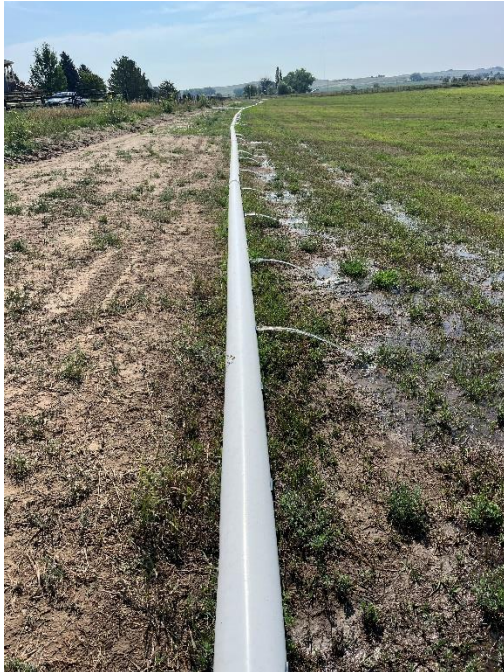
Photo 1, Gated pipe from irrigation project this summer, approx. 500ft long with approx. 2ft head pressure and every 3 rd gate open. Picture was during initial adjustment and not staked down yet.
