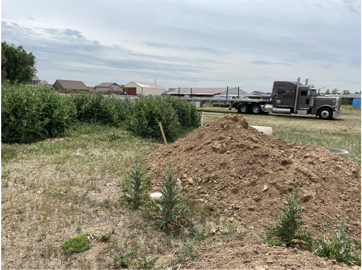
View towards soil treatment area
