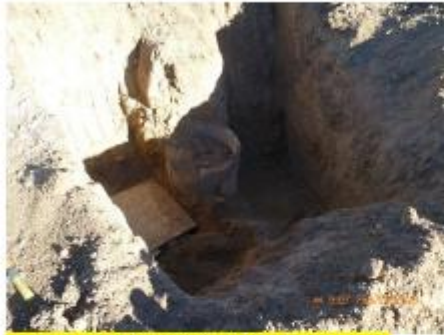
Secondary tank outlet – dug up previously
