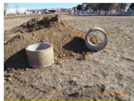
Risers removed from secondary tank outlet
