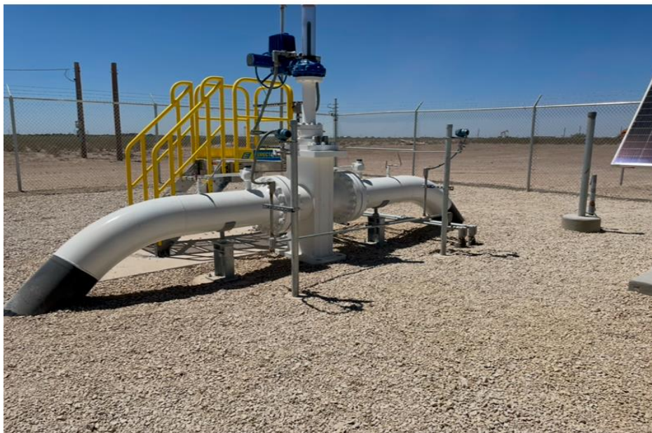
Rupture Mitigation Valve (RMV)
