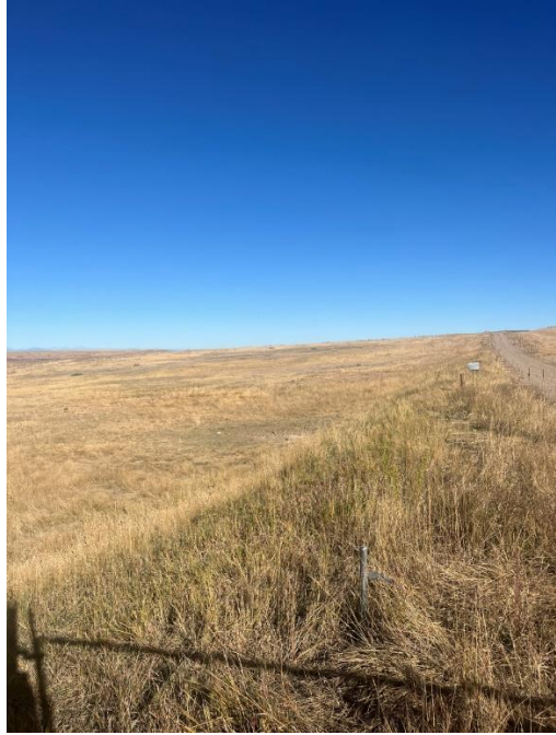
06. STR 691; view facing E. Grading of side slope from existing drive needed to access ROW
