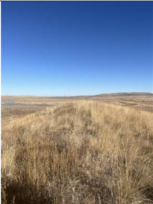
03. Berm adjacent to STR 696; view facing N.
