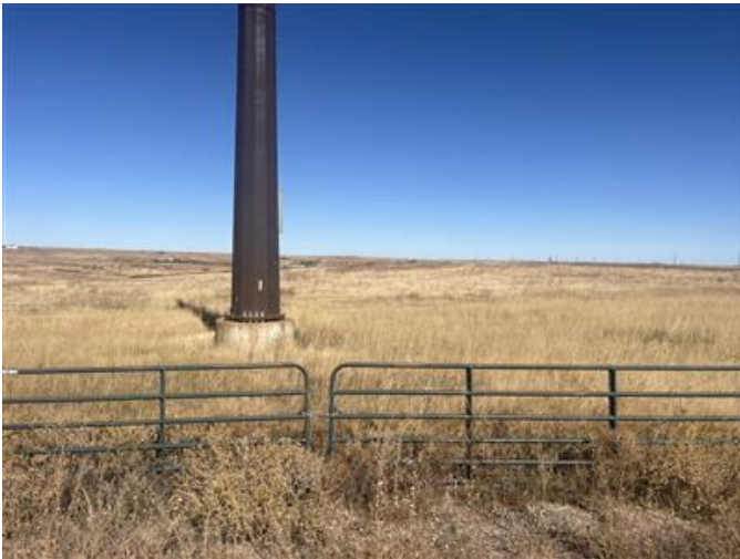
31. Access to STR 593; view facing N.
