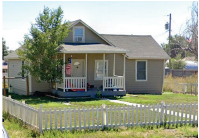
360 S. Sherman Street, constructed in 1939.
