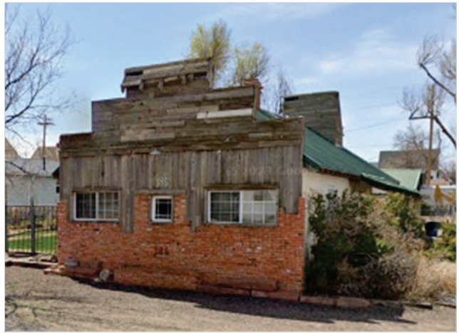
186 W. Front Street, constructed circa 1920 by George Kelley for his general merchandise store. By 1940, Kelley converted the building into his residence. Likely at this time, the original false front was shortened and modified to a "stepped" design.
