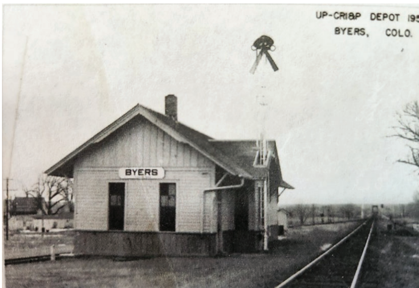
Byers Depot constructed circa 1900.
