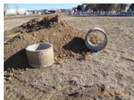
Risers removed from secondary tank outlet
