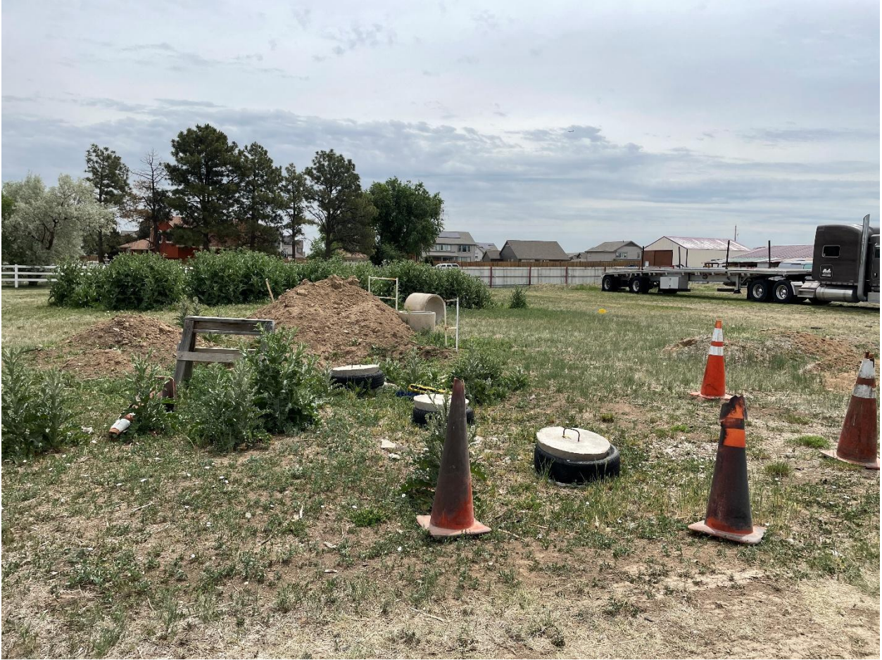
View of septic tank lids
