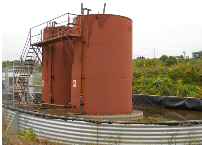
Storage tanks for produced water from natural gas drilling in the Marcellus Shale of Western Pennsylvania are surrounded by spill-containment structures. Storage tanks are one of the main sources of oil- and gas-field spills. Image credit: Doug Duncan, U.S. Geological Survey. 12
