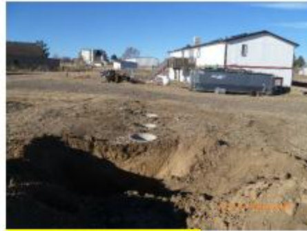
Tank to house facing northeast
