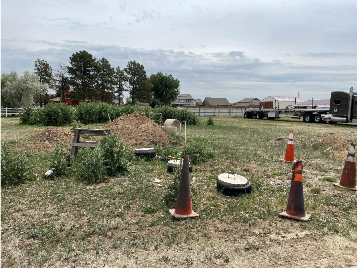
View of septic tank lids
