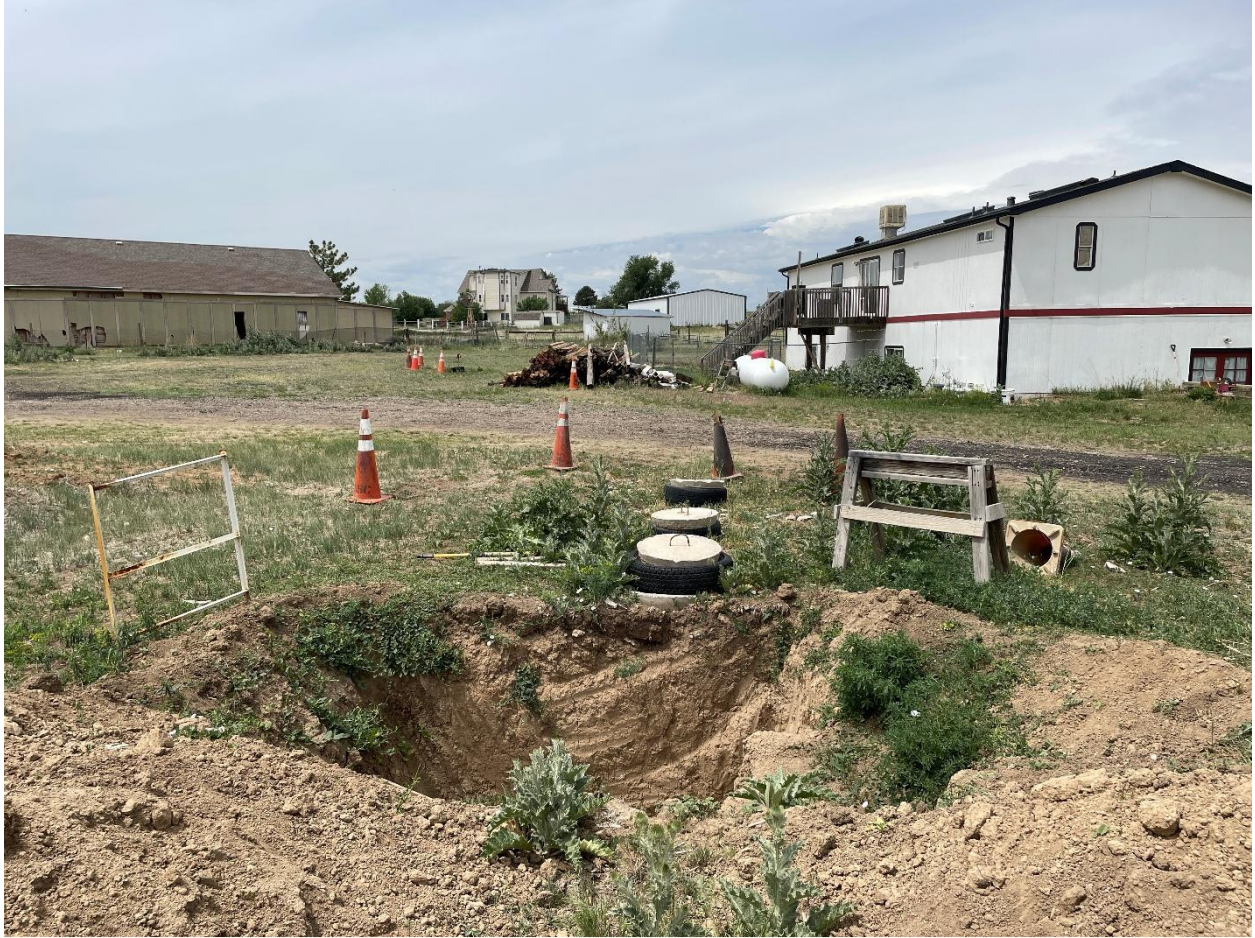
View of excavation
