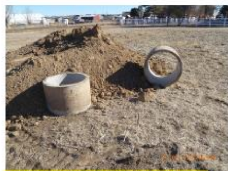
Risers removed from secondary tank outlet
