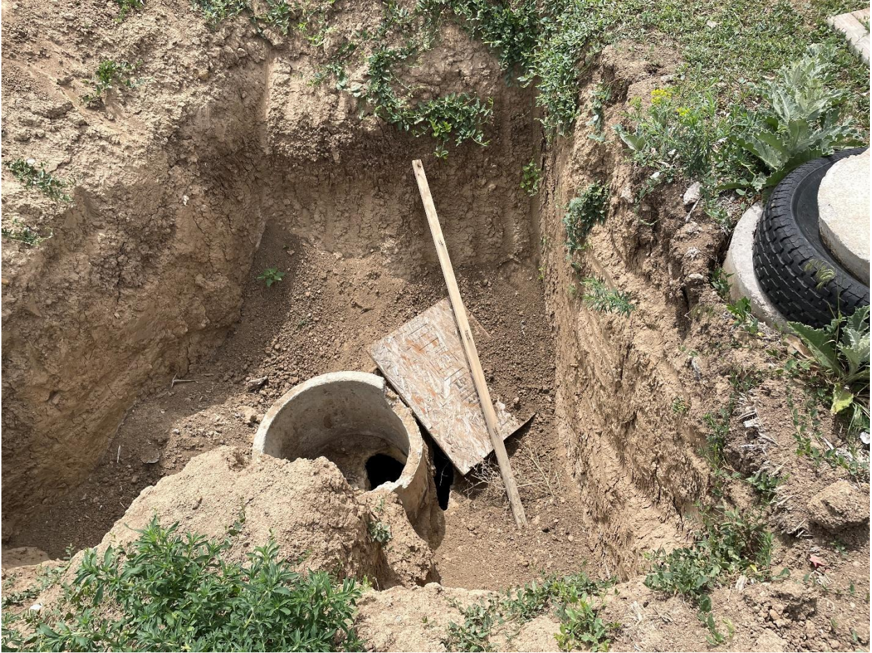
View of excavation
