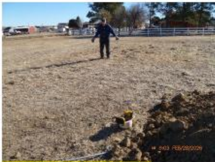
Diverter valve to STA 2 facing east
