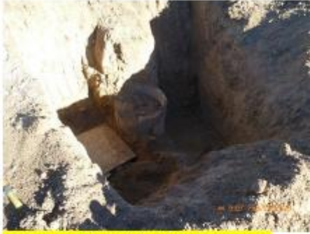
Secondary tank outlet – dug up previously
