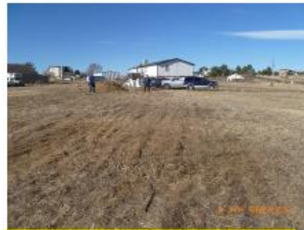
End of STA 2 back to diverter valve facing west
