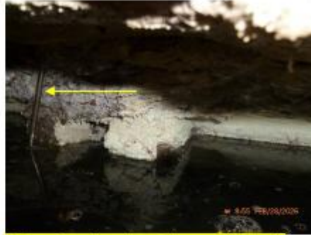
Probe through outlet wall – secondary tank
