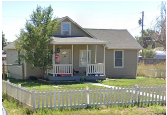
360 S. Sherman Street, constructed in 1939.
