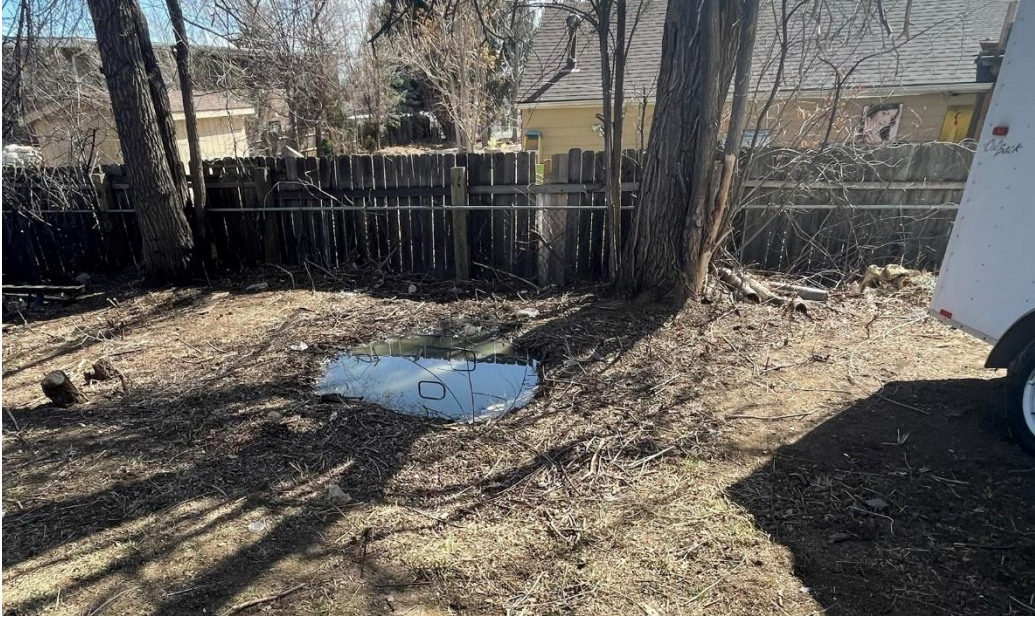
Photo of standing effluent approximately 45 feet from South side of home, looking South
