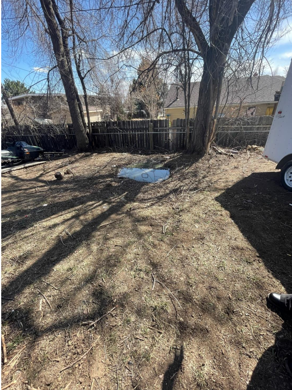
Full scale photo of standing effluent, showing neighboring fence line directly behind the tank (South)
