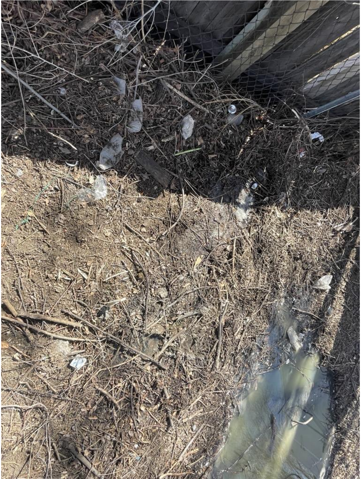
Photo showing proximity (approximately 5 feet) of surfacing effluent to the fence line. Photo angle is looking West
