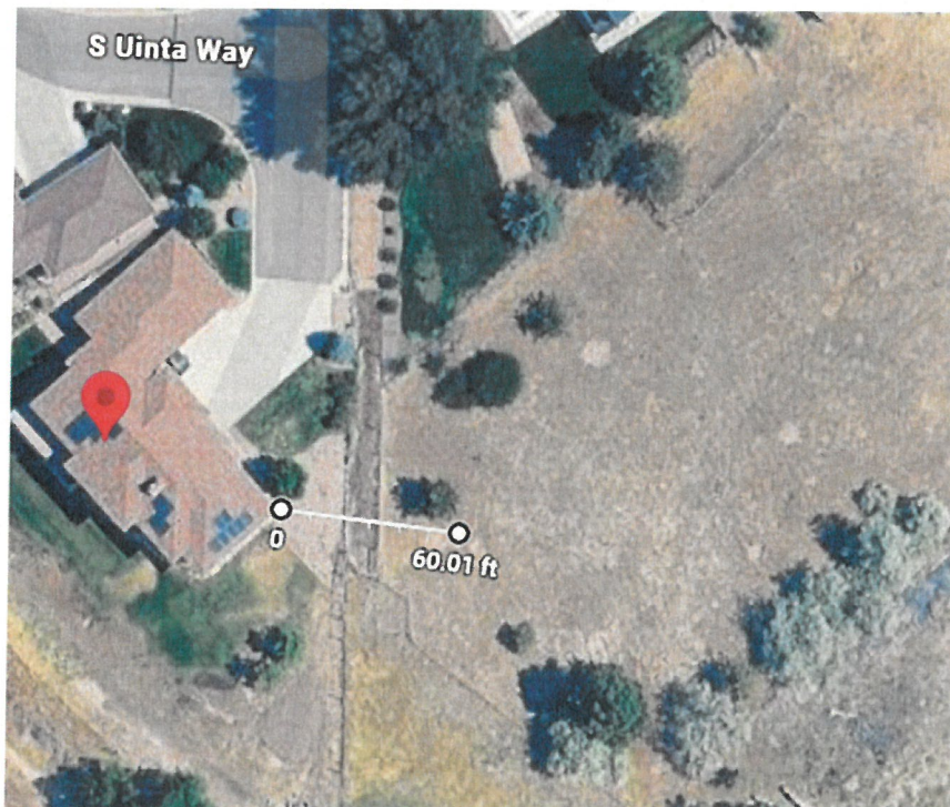
Figure 1: Areal Photo of Proposed Drainage Basin Area
