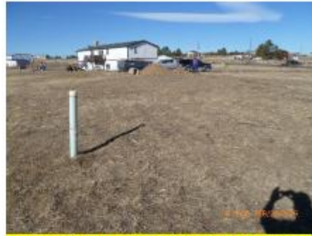
Back of STA 1 to diverter valve facing northwest
