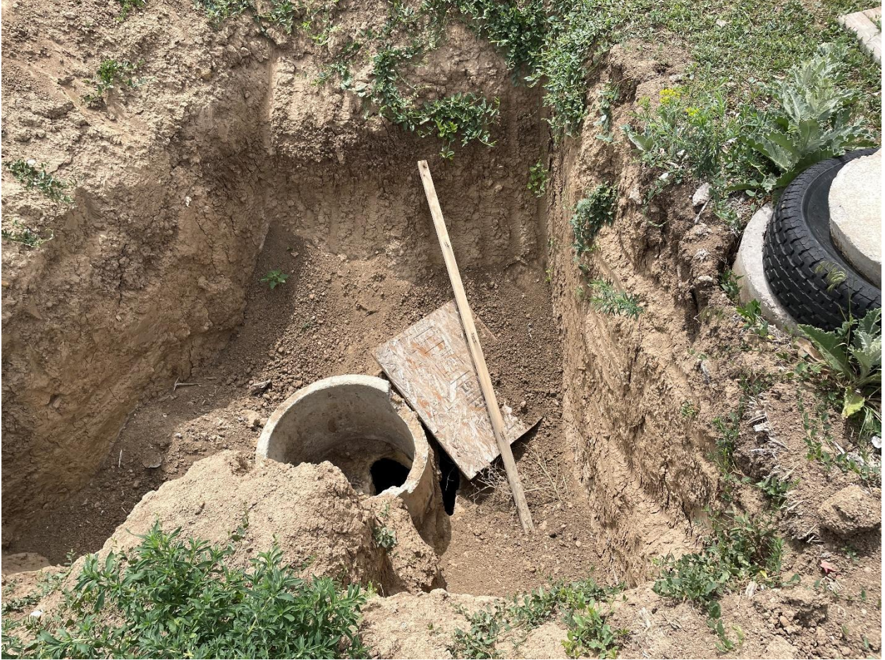
View of excavation
