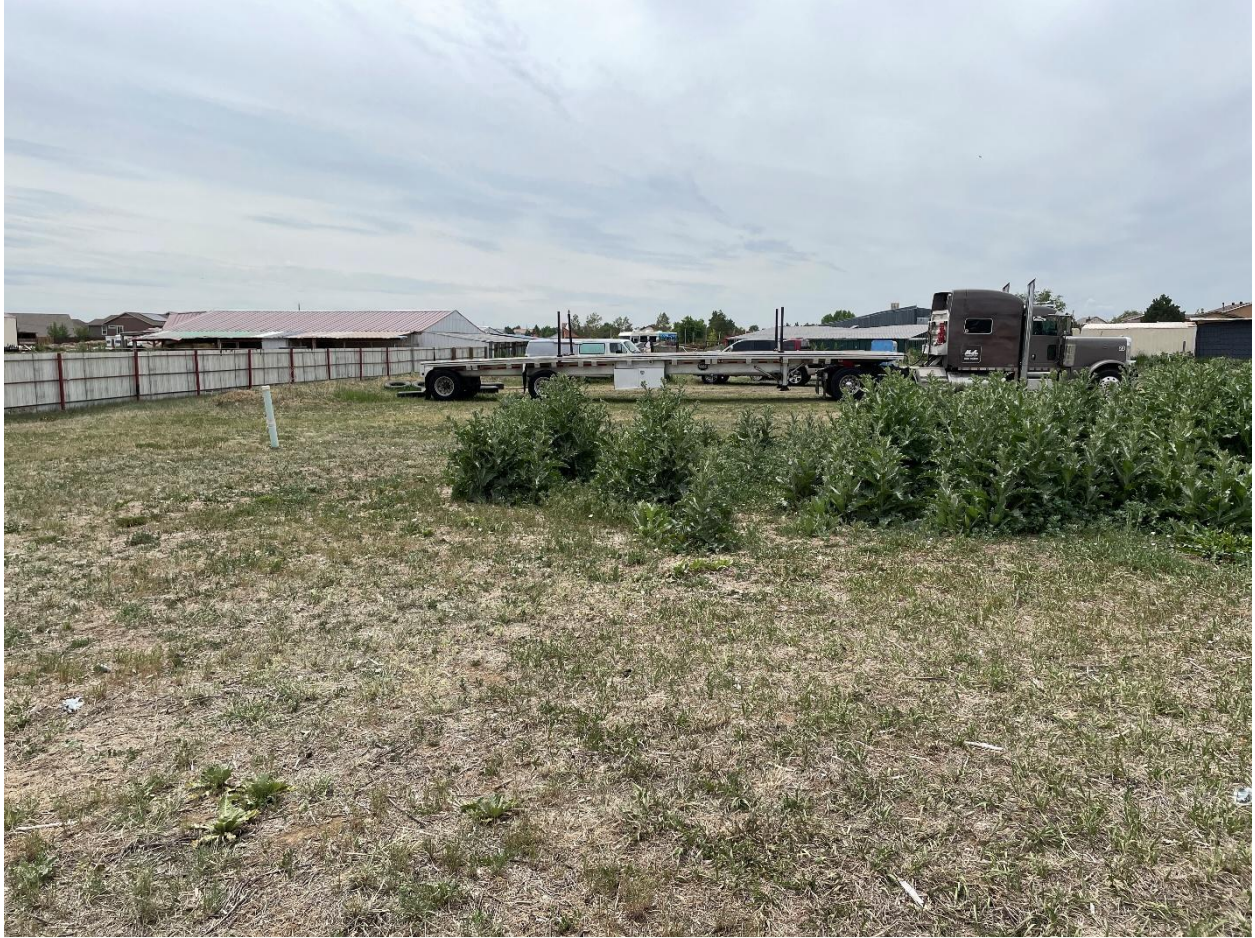
View of soil treatment area and observation port
