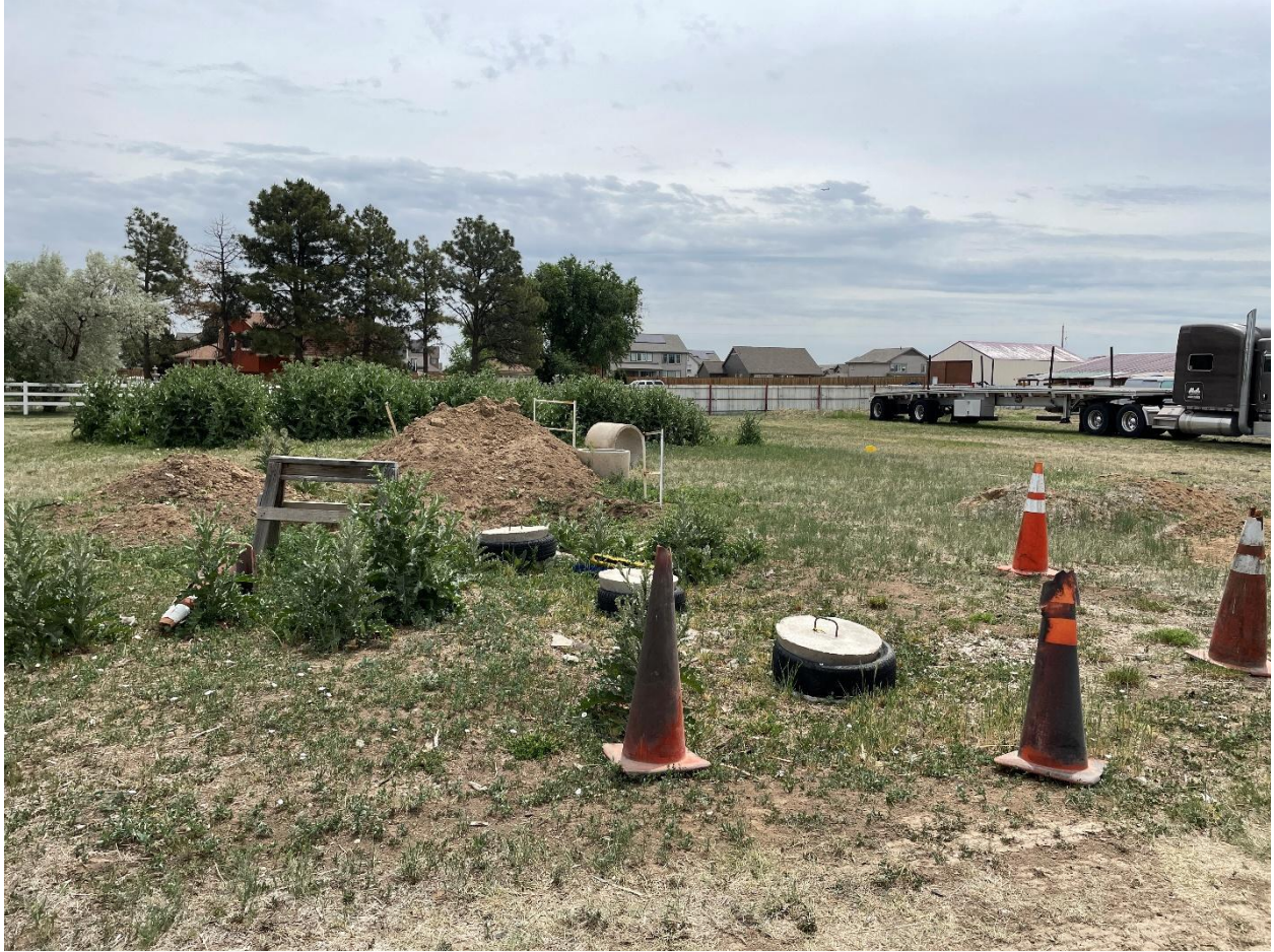
View of septic tank lids
