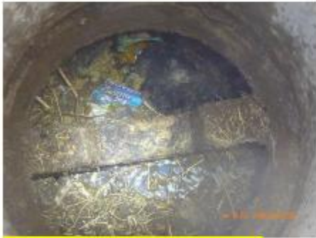
Inlet access port opening – primary tank
