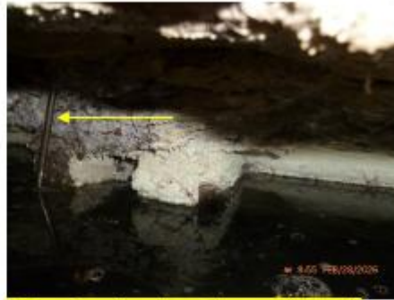
Probe through outlet wall – secondary tank
