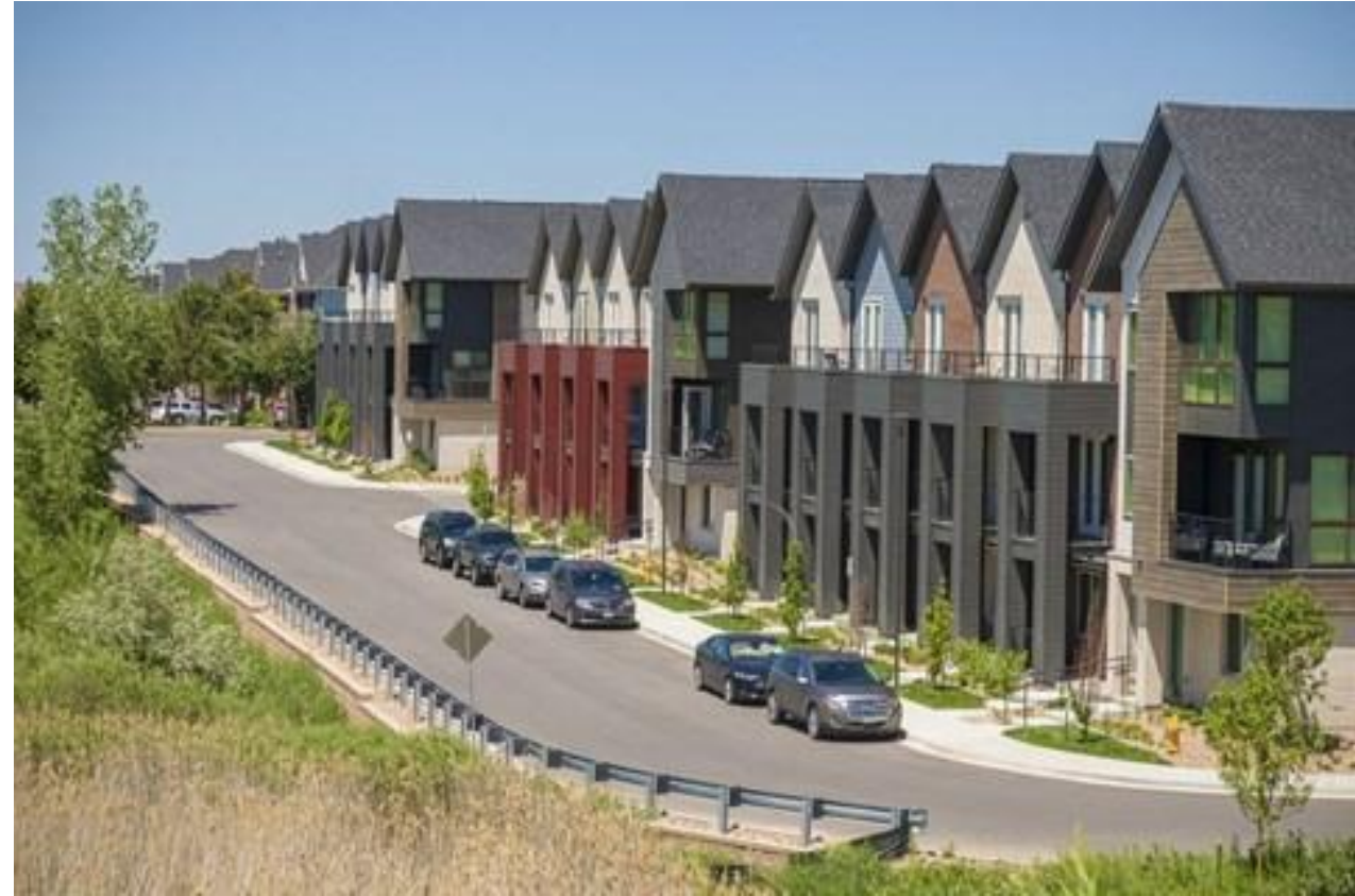
Dayton Station Townhomes north of subject property
