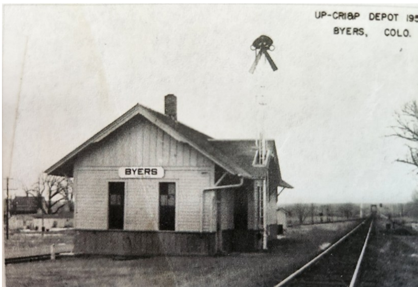
Byers Depot constructed circa 1900.
