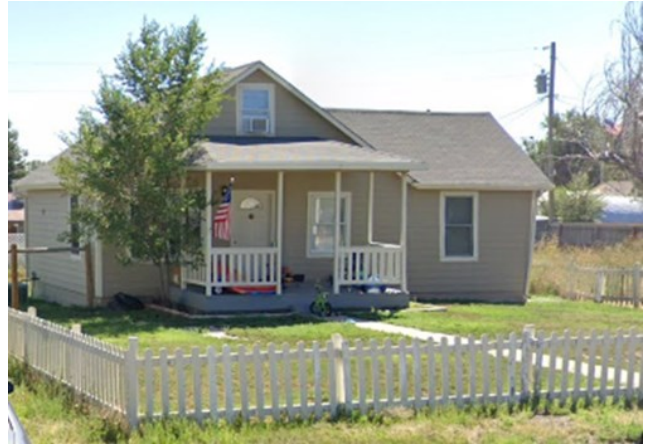
360 S. Sherman Street, constructed in 1939.
