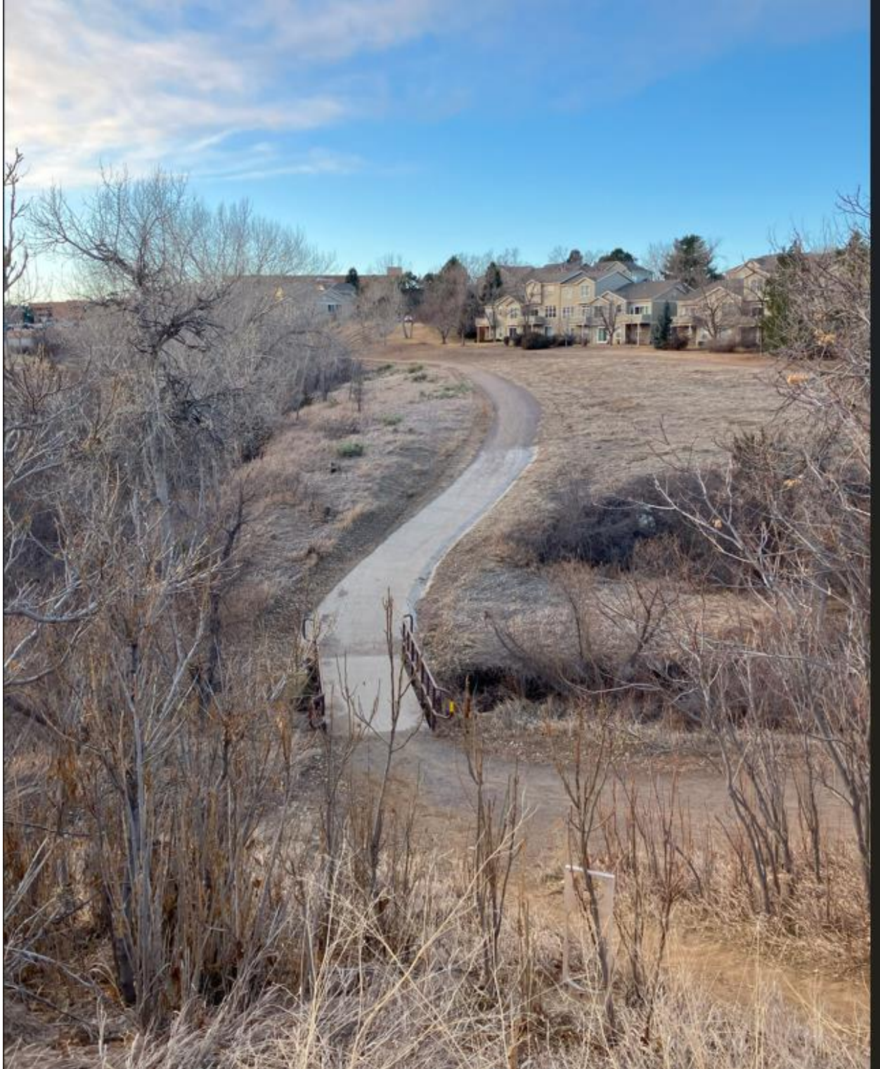
West Side – Lee Gulch Trail bridge crossing
