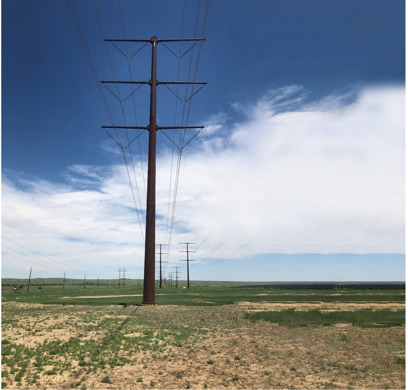
Representative Transmission Line
