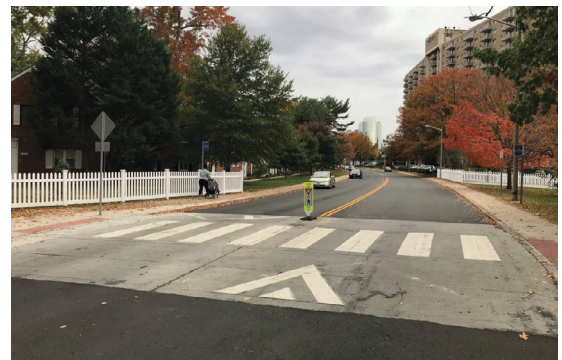
Raised Crosswalk, Alexandria, VA
