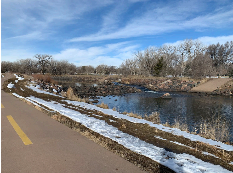
Drop structure 2. Angular riprap and unnatural appearance, and large vertical drop. Steep slopes in/out of water.
