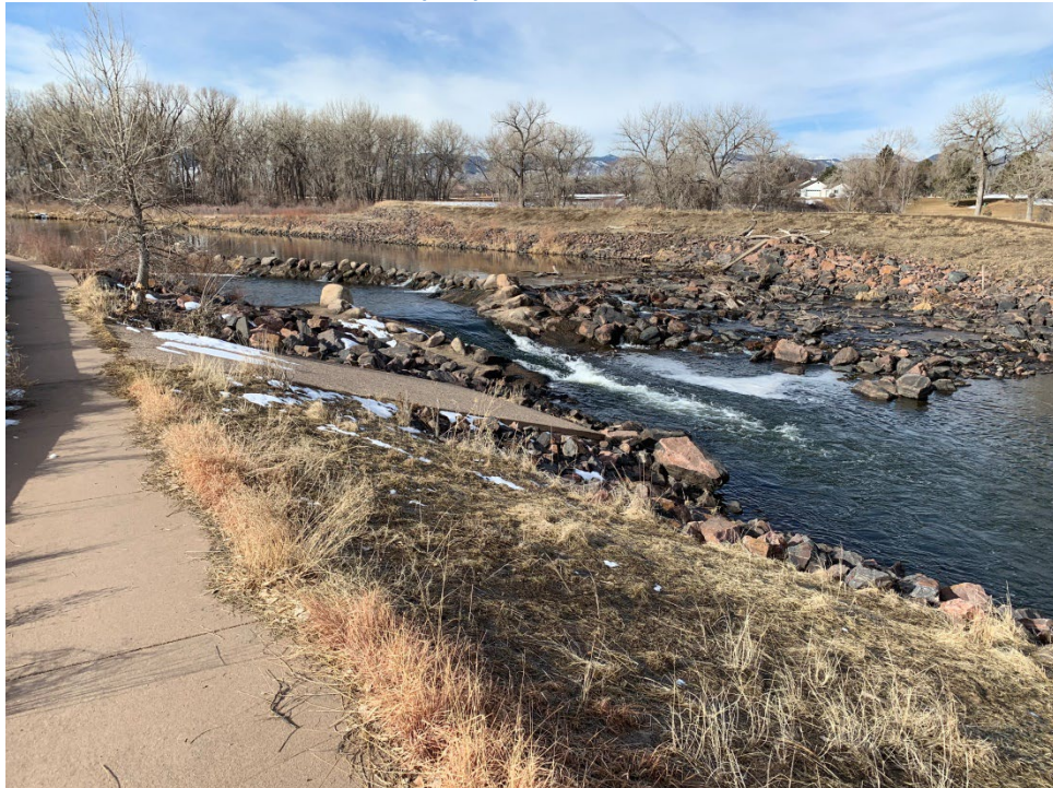
Drop structure 2. Angular riprap and unnatural appearance, and large vertical drop. Steep slopes in/out of water.
